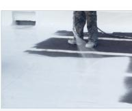
All protrusions in the roof were treated with a 3 course system (coating-fabric-coating) and received coating on the entire fixture. This ensured a watertight seal where the old system was vulnerable to leaks.
