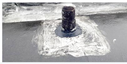
The previous roofing system, a smooth-surface built-up roof, had severe wear and tear around all protrusions and building edges. These areas were given a three-course silicone treatment of coating-fabric-coating to ensure a water-tight seal.
