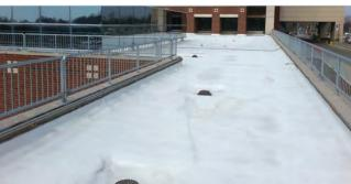
One of the most difficult aspects of this roofing project was the drainage. On top of requiring new slope, the roof had over 150 penetrations, most of these in the form of roof drains. Foam was the best tool available with regard to guiding water to the drains, and then creating a smooth, water-tight seal at the drains.
