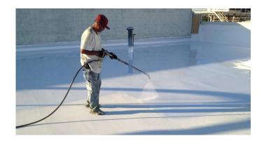
On vertical surfaces, ensure the material is not applied too thick as to cause runs or sags. At higher temperatures, the material will sag much easier than at lower temperatures.
