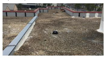
After the CLA thoroughly cleaned the roof, it was time to put down the primer. On most silicone jobs, primers aren't necessary. On gravel roofs, however, PM's P-160 is important due to the amounts of mini crevasses on the roof. The primer works its way into the cracks and crevasses of the gravel, offering the surface-leveling silicone stronger adhesion. On gravel-built up roofs it's always important to hit every gap.
