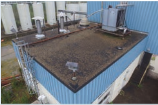
1. Original Gravel BUR roof surface
