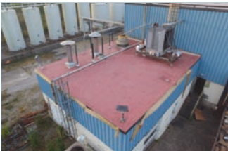
4. Apply SL 800 Surface Leveling Coating
