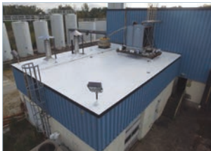
5. Apply HS 3200 Silicone Roof Coating
