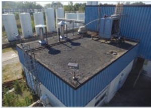
2. Remove loose rock
