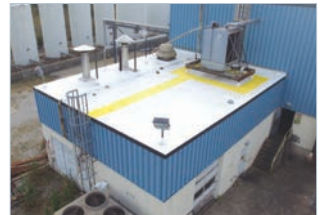
6. Apply Pro-Grip Walkway System (optional)
