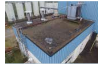
1. Original Gravel BUR roof surface
