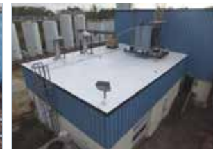
5. Apply HS 3200 Silicone Roof Coating
