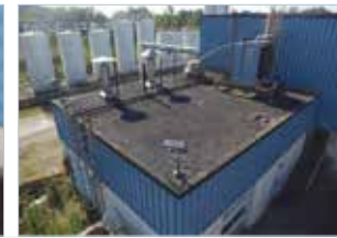
2. Remove loose rock
