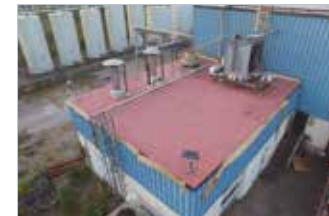
4. Apply SL 800 Surface Leveling Coating
