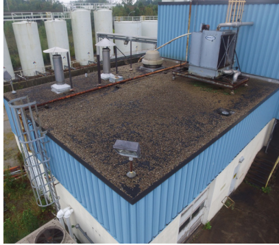
1. Original gravel BUR roof surface.
