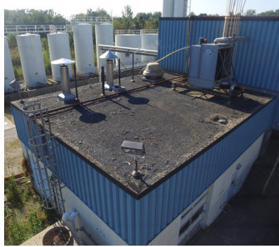
2. Remove loose rock.
