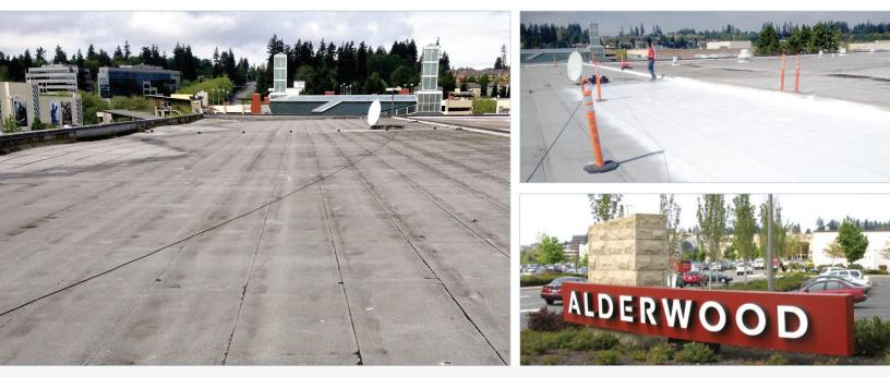
The Macy's roof in Lynnwood, Washington showed severe signs of deterioration and water damage. After patching and repair work was completed, the Progressive RCR process provided a waterproof, sustainable system that pleased Macy's facility management.
