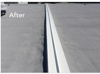
Because the roof had been ignored for so long, there was extensive damage to the roofing surface that was not repaired. Not only the foam, but many of the metal features of the roof were in poor condition. Once the old gravel and foam were removed from the roof, all metal features, such as the expansion joint pictured above, were replaced with new metal. The new foam was then installed around the metal features, which provided a completely new roof surface.
