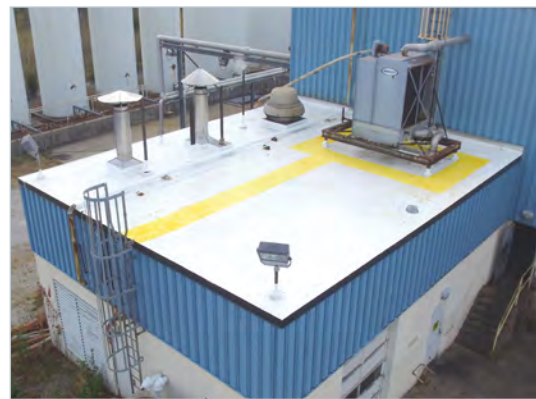
6. Apply Pro-Grip Walkway System (optional)
