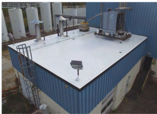
5. Apply HS 3200 Silicone Roof Coating
