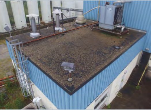
1. Original Gravel BUR roof surface
