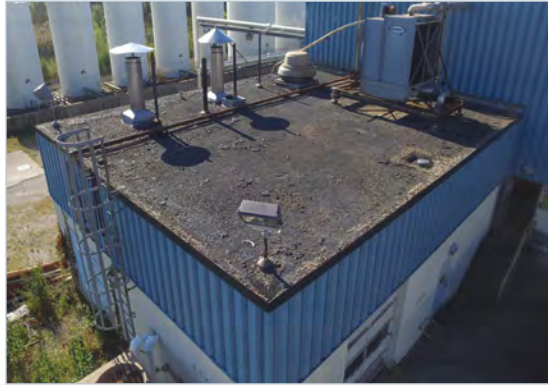
2. Remove loose rock
