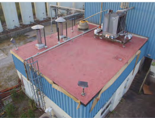
4. Apply SL 800 Surface Leveling Coating
