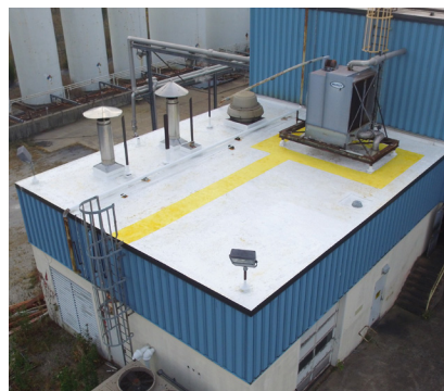
6. Apply Pro-Grip Walkway System (optional)
