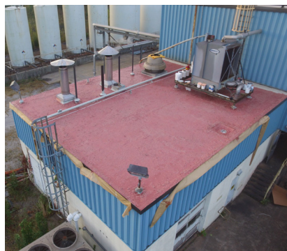
4. Apply SL 800 Surface Leveling Coating
