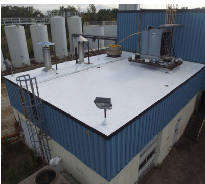
5. Apply HS 3200 Silicone Roof Coating
