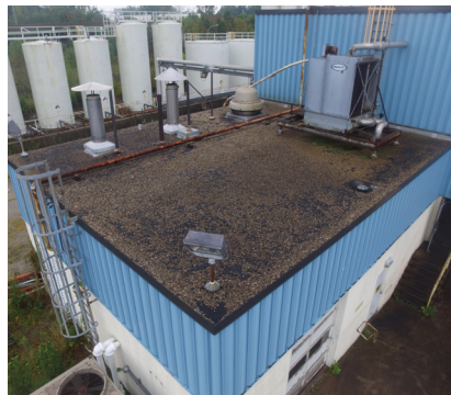
1. Original Gravel BUR roof surface
